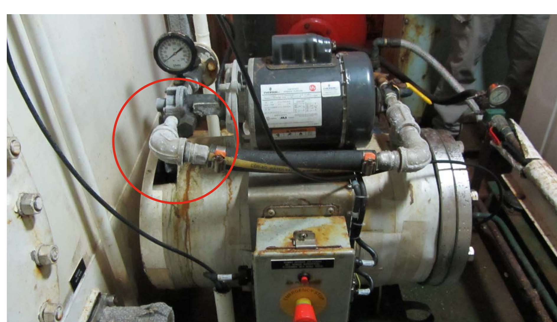
the water to flow constantly; this pump is installed inside the hold of the vessel, mainly to prevent the direct contact of the sensor with the ice that is frequently in work areas. Nevertheless, the adverse weather conditions in
