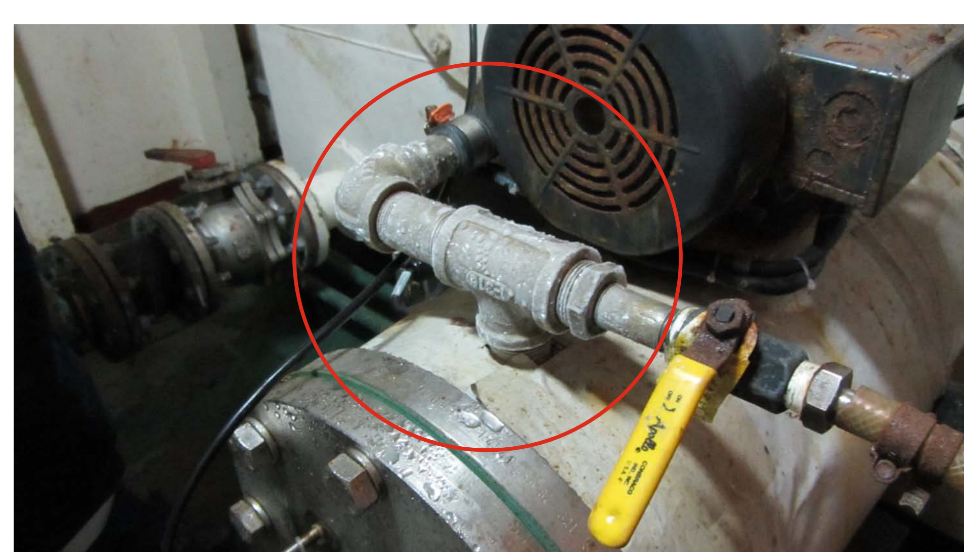
One of the major components of the multibeam system is the surface sound velocity sensor (SSV), whose aim is to monitor the sound velocity to 6.35 m depth every 2 seconds. This sensor is installed within a pump, which allows
